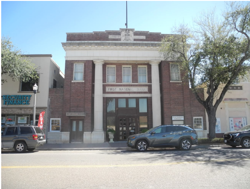
Photo 15 – former First National Bank 334 S. Texas Ave.
