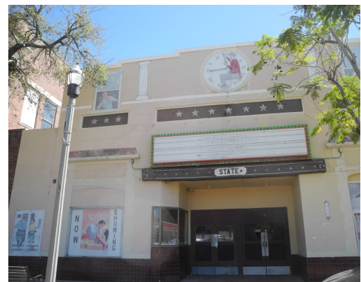
Photo 49 – State Theater 344 S. Texas Ave.
